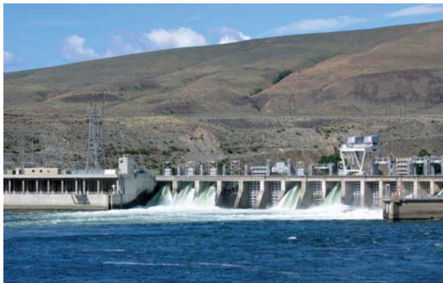
Hydroelectric dam in the Northwest
